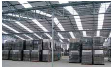
Transparent roof project to reduce lighting usage
