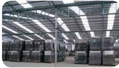
Transparent roof project to reduce lighting usage.
